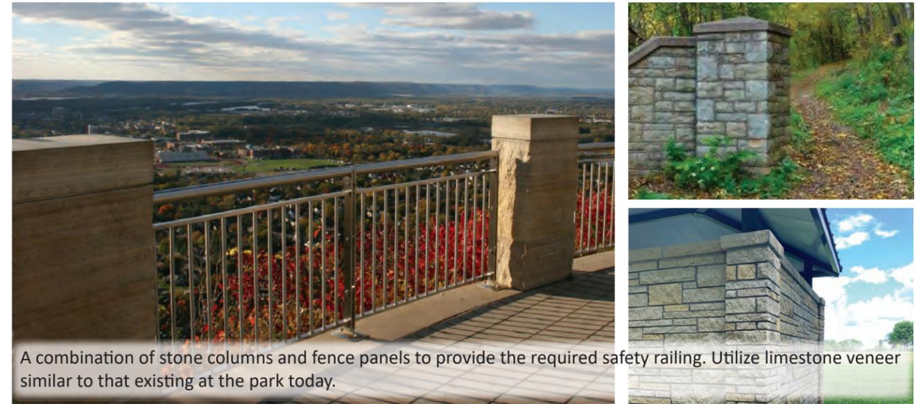
A combination of stone columns and fence panels to provide the required safety railing. Utilize limestone veneer similar to that existing at the park today.
